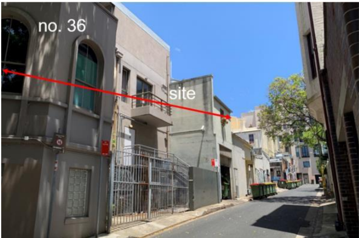
Figure 8: Rear of subject site as viewed from Mansion Lane
