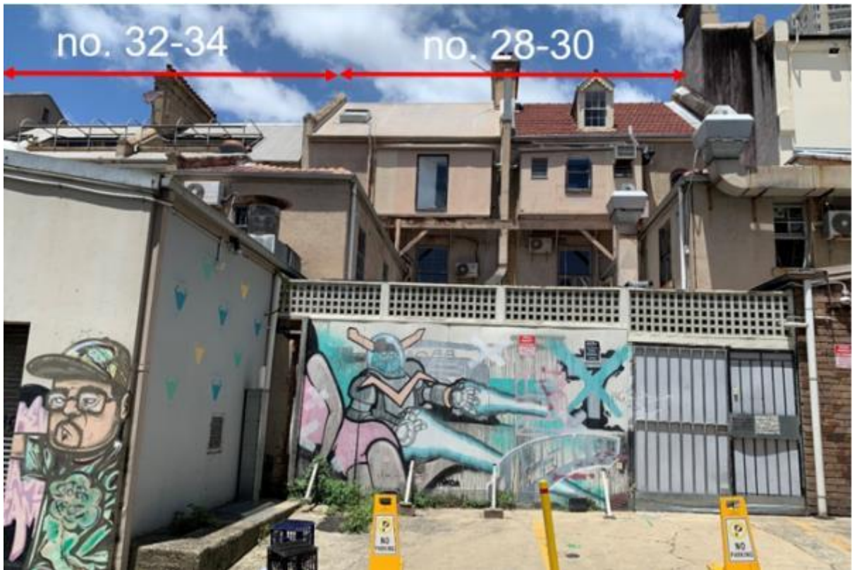
Figure 9: Rear of subject site as viewed from Mansion Lane
