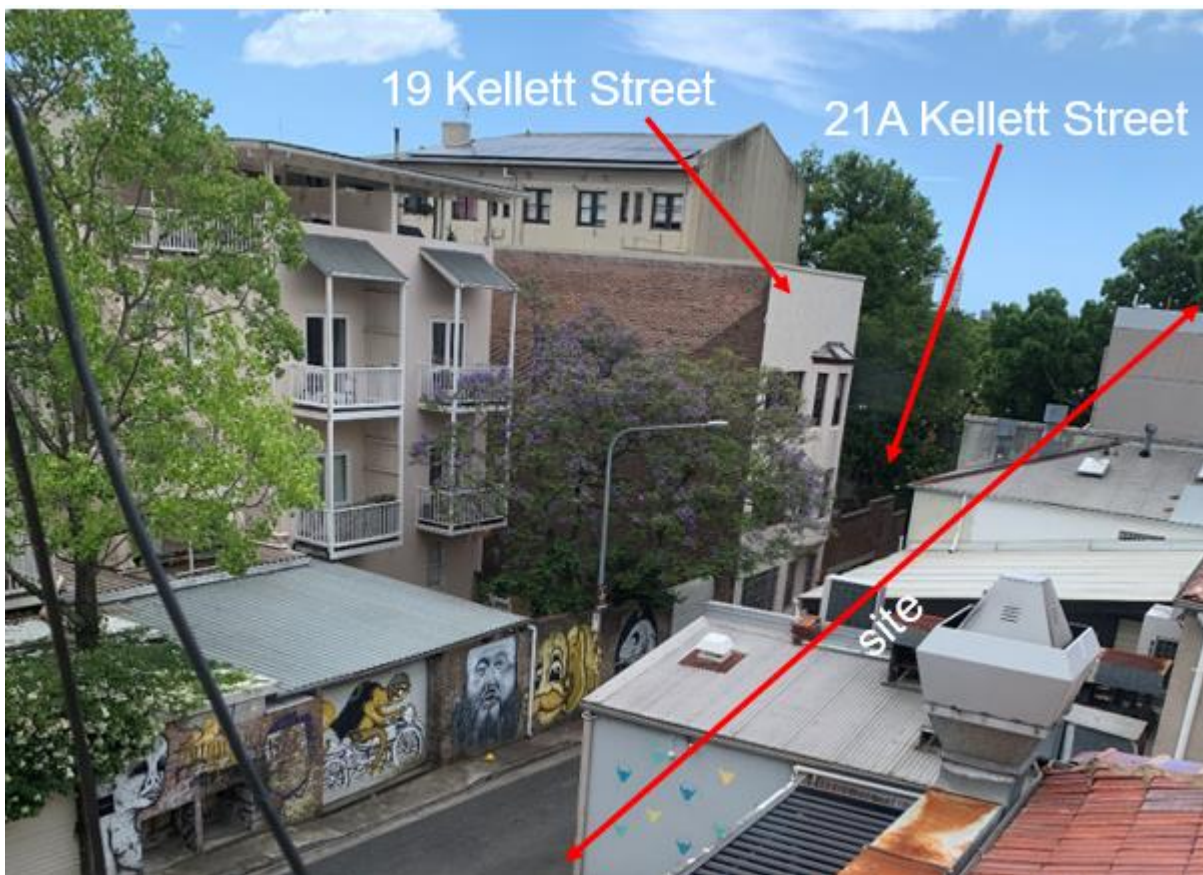
Figure 55: Existing development on the northern side of Mansion Lane
